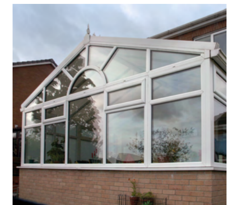
WHITE CONSERVATORY WITH SUNBURST DESIGN AND POLYCARBONATE ROOF
